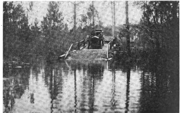
ONLY DEEPEST PARTS OF THE RIVERS ARE BRIDGED.
